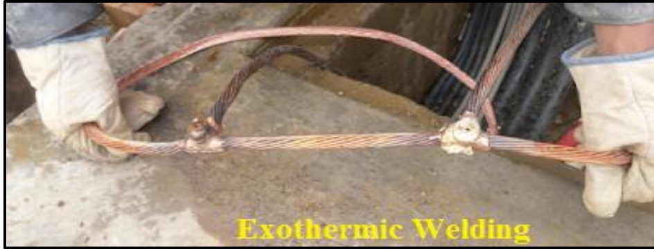
Exothermic Welding
