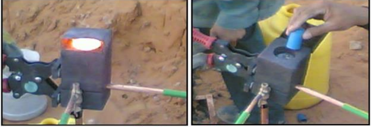
Exothermic Welding
